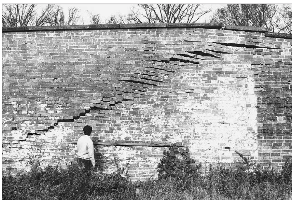
Figure 1. Reactivation of a fault generated a 0.3m high fault scarp and caused severe damage to a 5m high brick wall at Eastwood Hall. The date of reactivation is not known, but was probably in the 1960s. This section of wall has been demolished, but evidence of further fault reactivation was visible on an opposing wall in May 2000.
