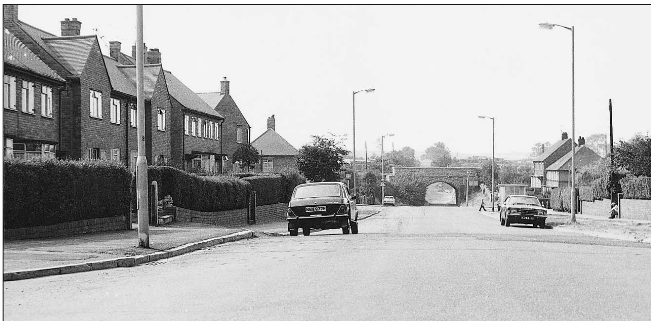
Figure 6. Reactivation of a fault in 1976, generated a scarp 0.5m high that caused moderate damage to Vale Road, Mansfield.
